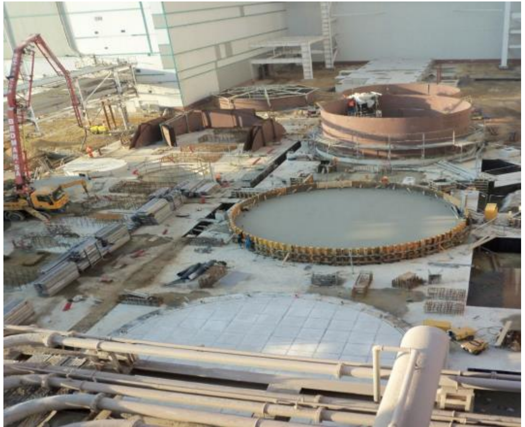
Foundations for absorbers, pump stations and other facilities
