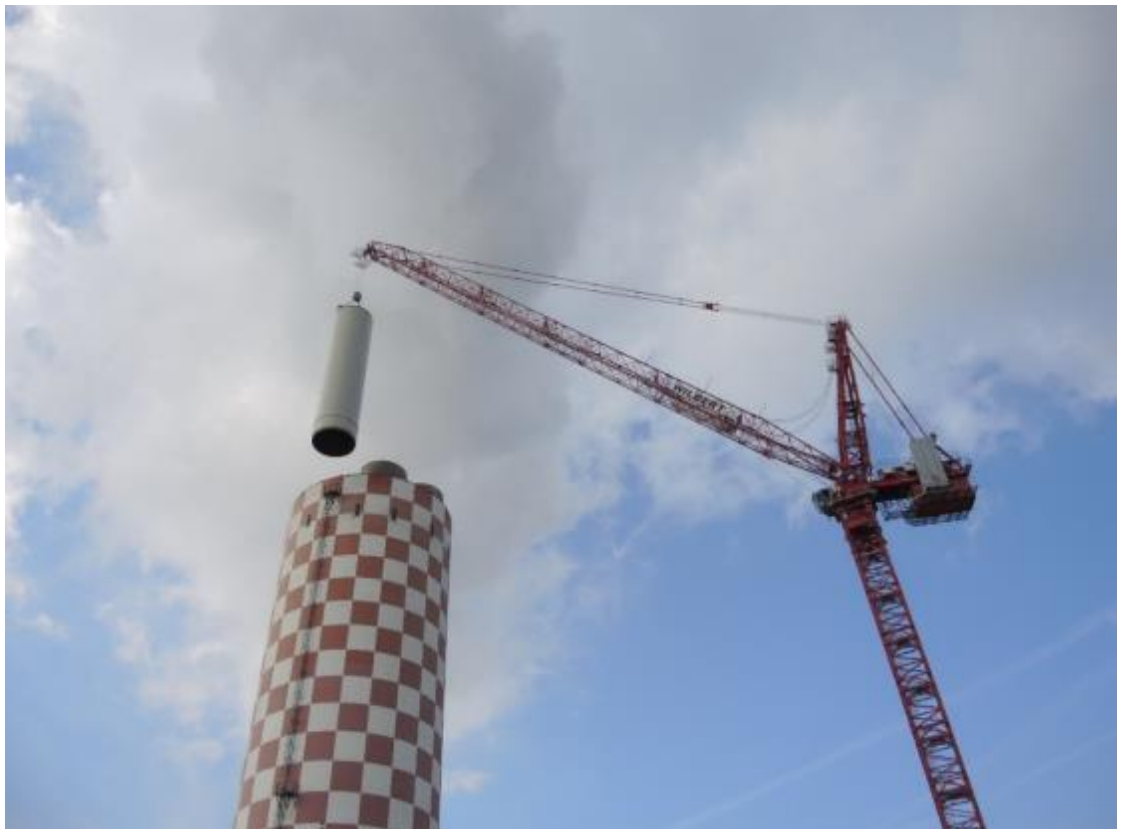
Adaptation of the last six-conduit chimney draught
