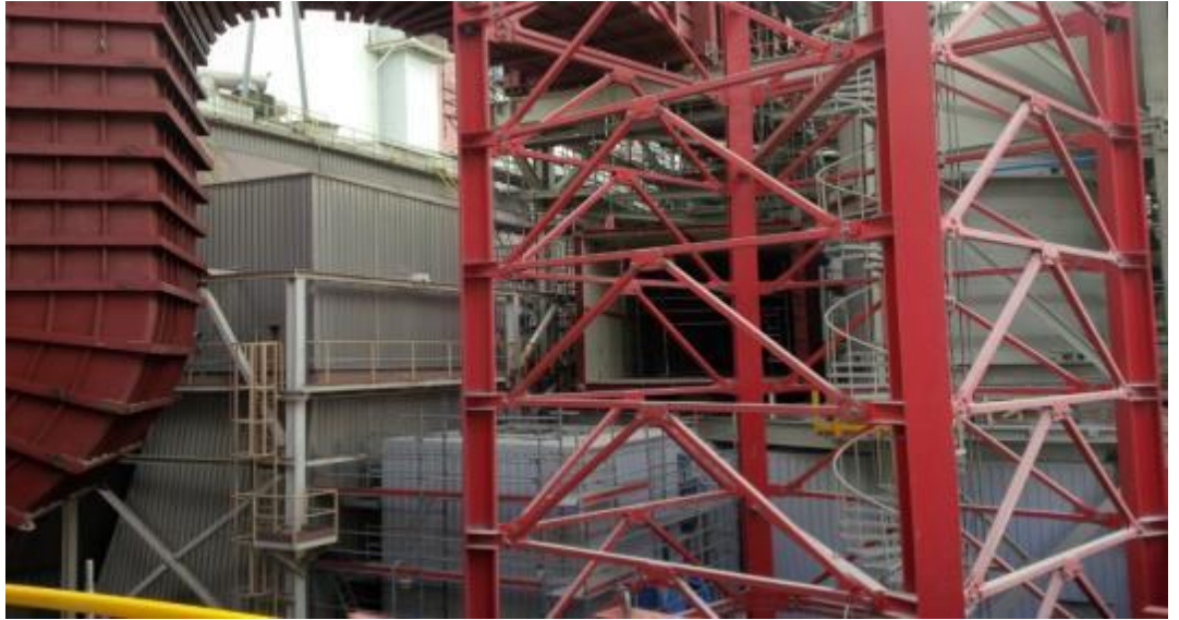
Assembly and start-up of flue gas fan for unit no. 5
