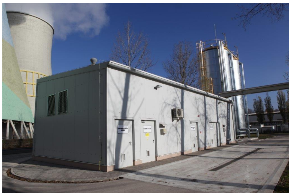
Reagent unloading and storage station
