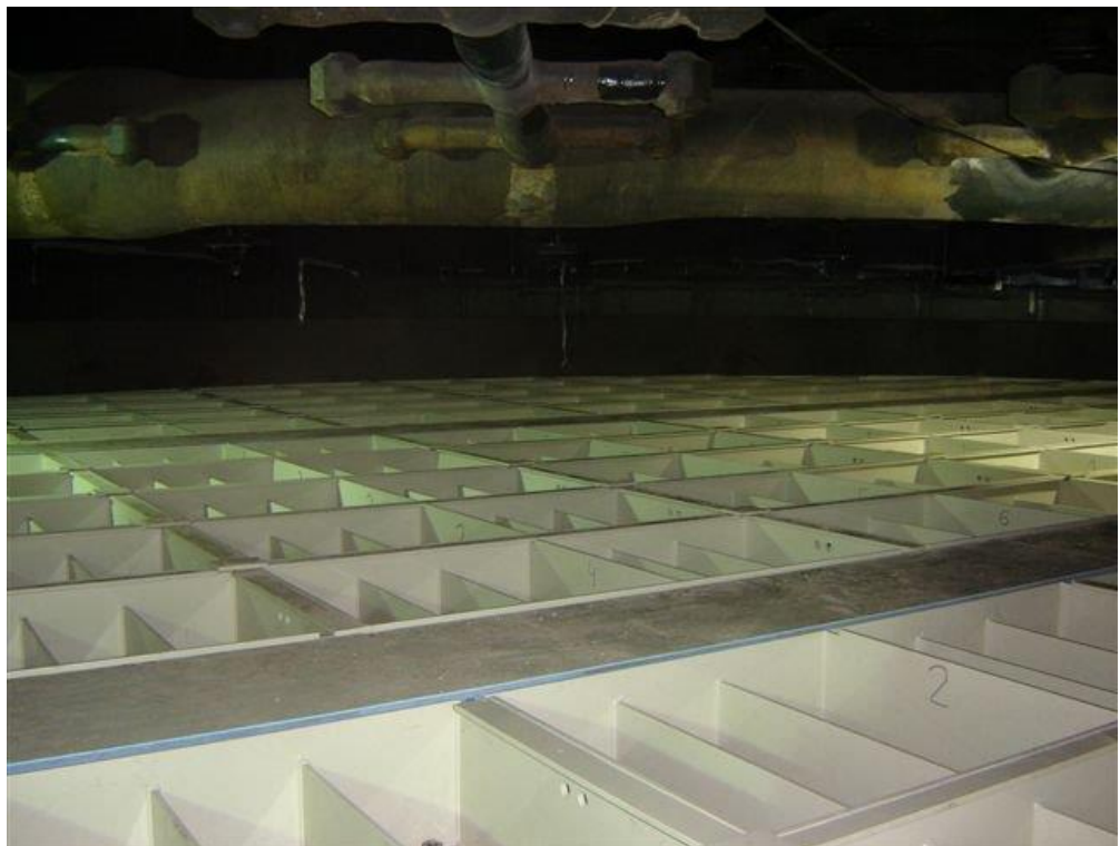
Sieve plate - sprinkling level
